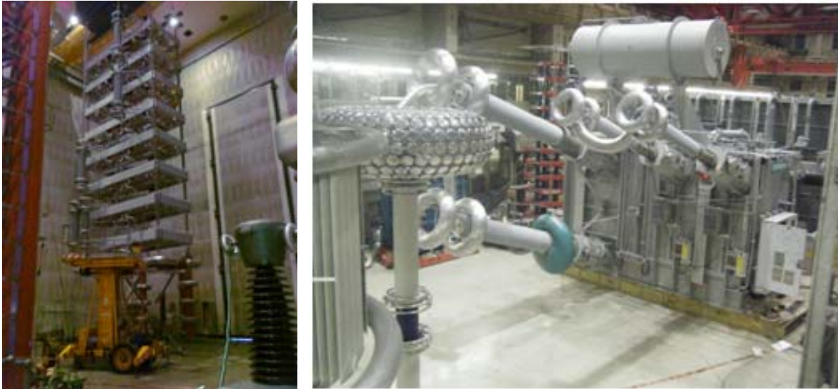
Figure 4: Thyristor quadruple valve impulse testing at University of Karlsruhe, Germany (left) and converter transformer factory impulse testing at Nurnberg (right)
