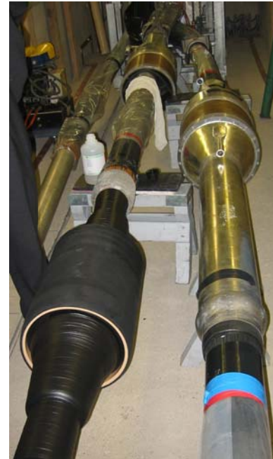
Figure 2.6: XLP Cable Jointing in Progress
