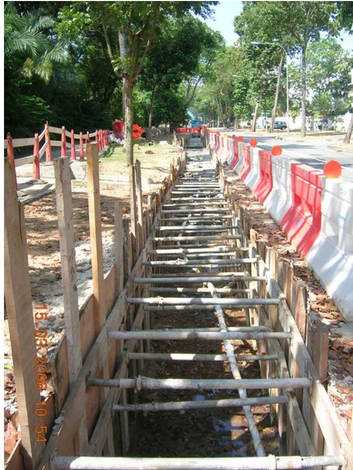
Figure 2.8: Excavated Cable Trench with Existing Utility Service Structure
