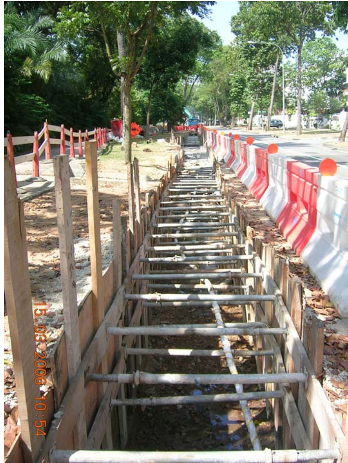
Figure 2.8 Excavational Cable Trench with Existing Utility Service Structure
