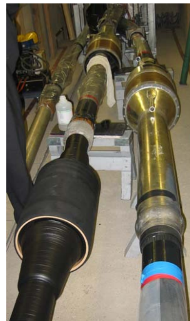
Figure 2.6 XLP Cable Jointing in Progress
