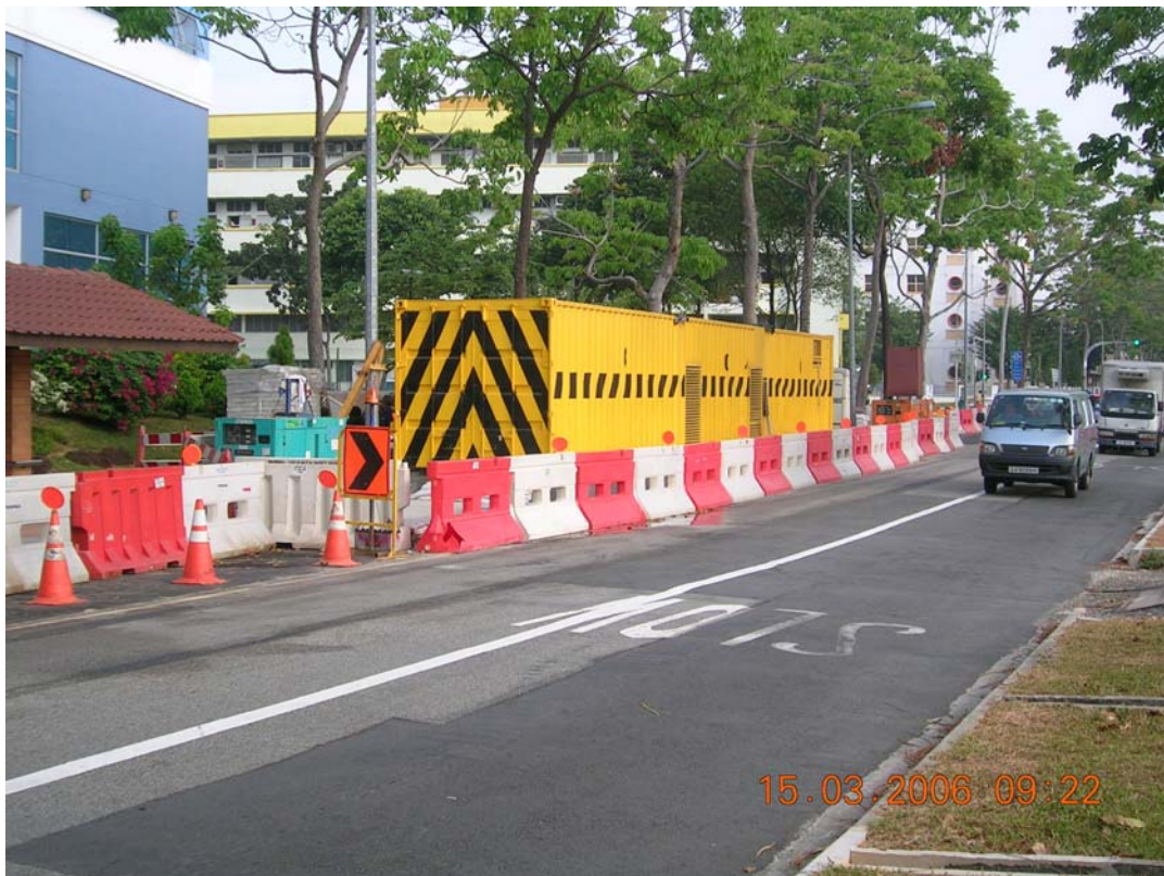
Figure 2.9 A Joint Bay Enclosure During the Construction Stage
